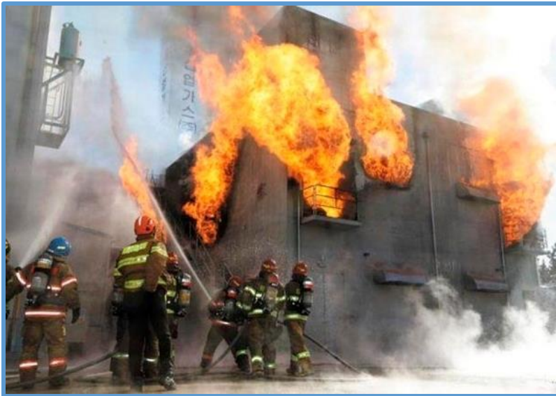
ESS Station in South Korea Lithium battery fire
